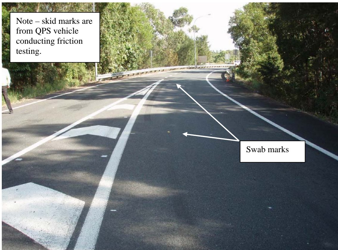
Photo 6 – Reverse view along ramp
